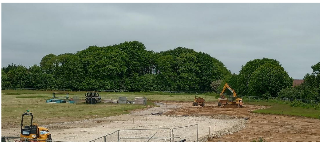
Grouting mats are being installed to the bottom of the image with top soil stripping occurring at the top.
