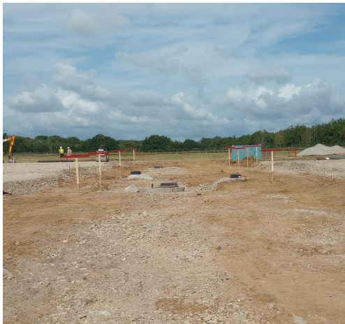
Street 2—drainage work complete, road formation to start
